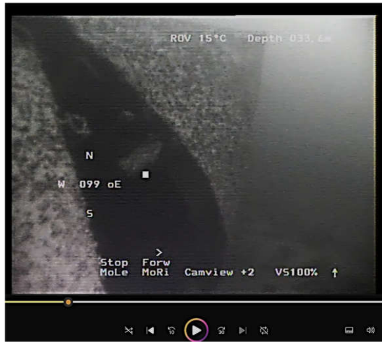
Fig. 5 Large crack in the sheathing
